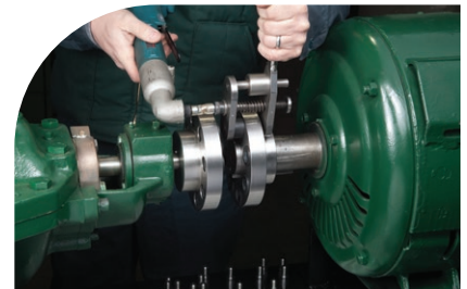
Installation of bushings using tool and battery operated angle ratchet wrench
